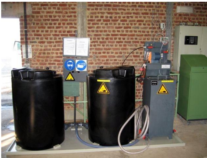
For municipal water, GO 2 TM concentrate is pumped from 1,000 liter tanks into the drinking water system. No dangerous generators or specially secured area's are necessary.
